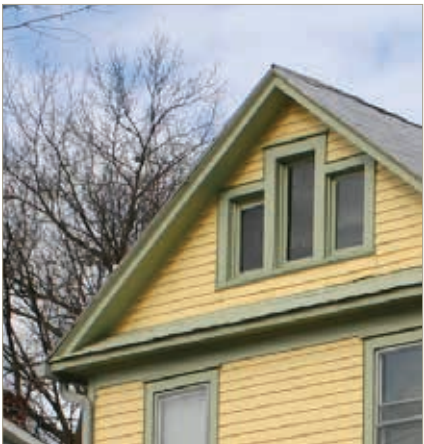
Cornice Fully Returned
