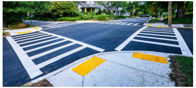
High-visibility crosswalks, ADA ramps and Speed Humps were installed throughout the City as part of the SS4A Project.
